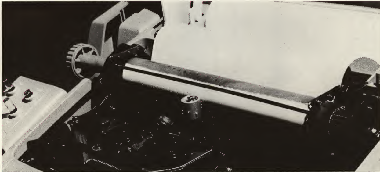
Braille Head and Modified Platen
